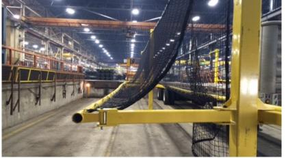
Pivoting (cantilever) system that does not attach to the trailer at all; instead, it swings in and out to allow for quick setup and eliminates the risk of a driver leaving with the nets still attached.
